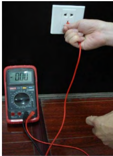
Appendix Figure 7-5 Check earth cable connection
