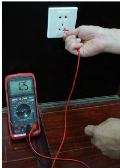
Appendix Figure 7-6 Check live cable connection
